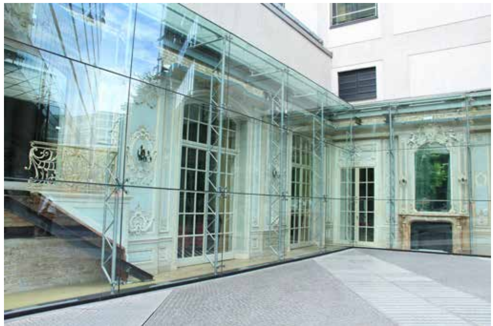
Hotel Esplanade Remains Under a Glass Cover, integrated into the Sony Centre. Photograph by Fred Romero, Paris, France, 2016. https://commons.wikimedia.org/wiki/File:Berlin_-_Hotel_Esplanade_remains_in_Sony_Center.jpg CCBY 2.0
